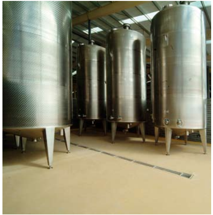
Sikafloor® 20 Purcem meets Health and Safety requirements at Quinn Glass
