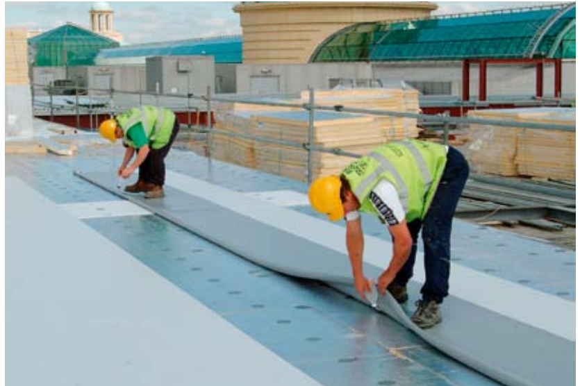
Sika-Trocral type S being applied to the Trafford Centre, Manchester
