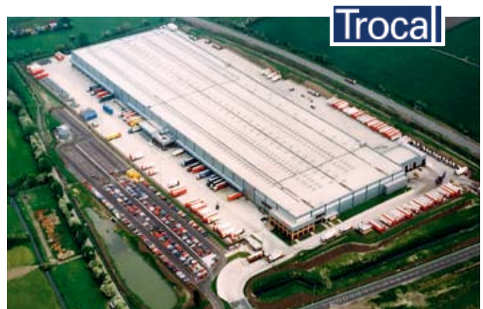
Tesco distribution centre at Magor, South Wales fitted with 57,000 square metres of Sika-Trocal type S fifteen years ago
